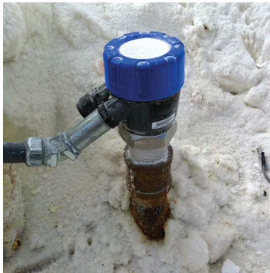
Tek-Flex 4100A with 1½" NPT mounting in liquids, slurries or solids applications.
